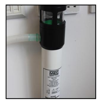
This picture shows one of the passive systems which relies on external air passing over the outlet tube to provide negative pressure and suction out the waste gases.
